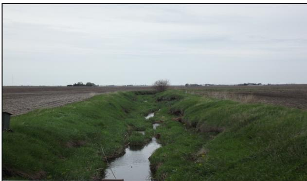
**Figure 1. Traditional agricultural ditch experiencing severe bank erosion and channel filling. The ditch itself is trying to establish a lower lying floodplain bench by undercutting its ditch banks and allowing them to fall into the wide channel bottom. (Photo Courtesy-The Nature Conservancy)**
