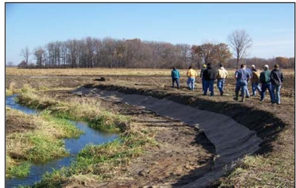
**Figure 2. A constructed 2-Stage Ditch establishes a stable low-lying bench along the main channel. This allows for the effective conveyance of high and low storm flows, increased flood storage, and various water quality and environmental benefits. (Photo Courtesy-The Nature Conservancy)**
